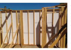
Allen chose to have LP FlameBlock sheathing installed as a part of the code-compliant U350 assembly in hopes that it would simplify the assembly process for his volunteers. He also wanted to avoid any safety hazards that a traditional shaft assembly wall may pose due to the complexity of the construction.
